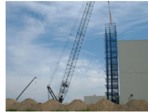
Begin Rack Erection
