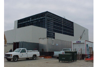
Complete Siding and Roofing
